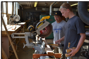
Students Max Nelms & Brody Griffin preparing the materials to build the stage.
